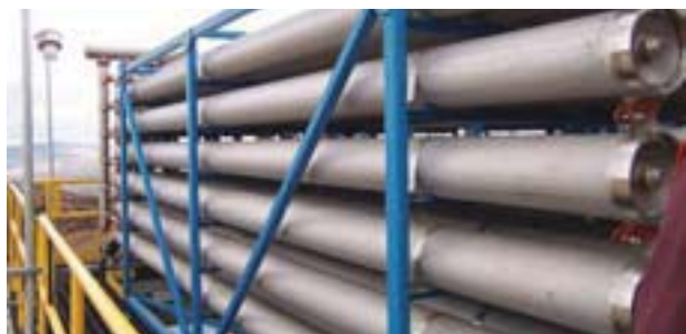
An engineered membrane system similar to the one pictured above recovered 2.5 million gallons of clean water and 28,000 pounds of copper each day at an open pit copper mine in Mexico. The custom designed treatment system increased copper production 14 percent by recovering copper otherwise lost in the mine wastewater.
